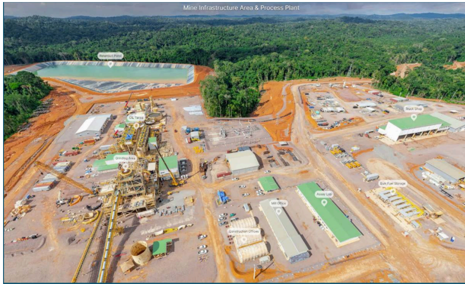
Figure 1 – Mine Infrastructure Area and Process Plant Progress
